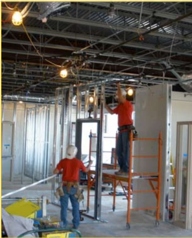
New SAMI office under construction.
